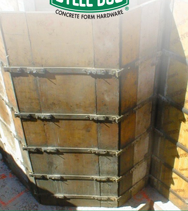
CC-45s Used on Bay Window Corners
